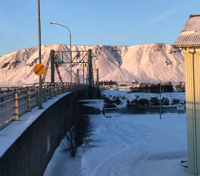
The bridge over Ölfusá river is over 70 years old and carries a heavy traffic load. Photo: Hjördis Rut Sigurjonsdottir
