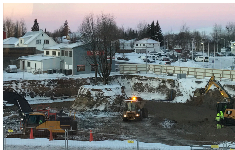
Not everything will be new in the new downtown area. The tree in the middle of this picture has been left in place, despite the heavy construction work. Photos: Hjördis Rut Sigurjonsdottir
