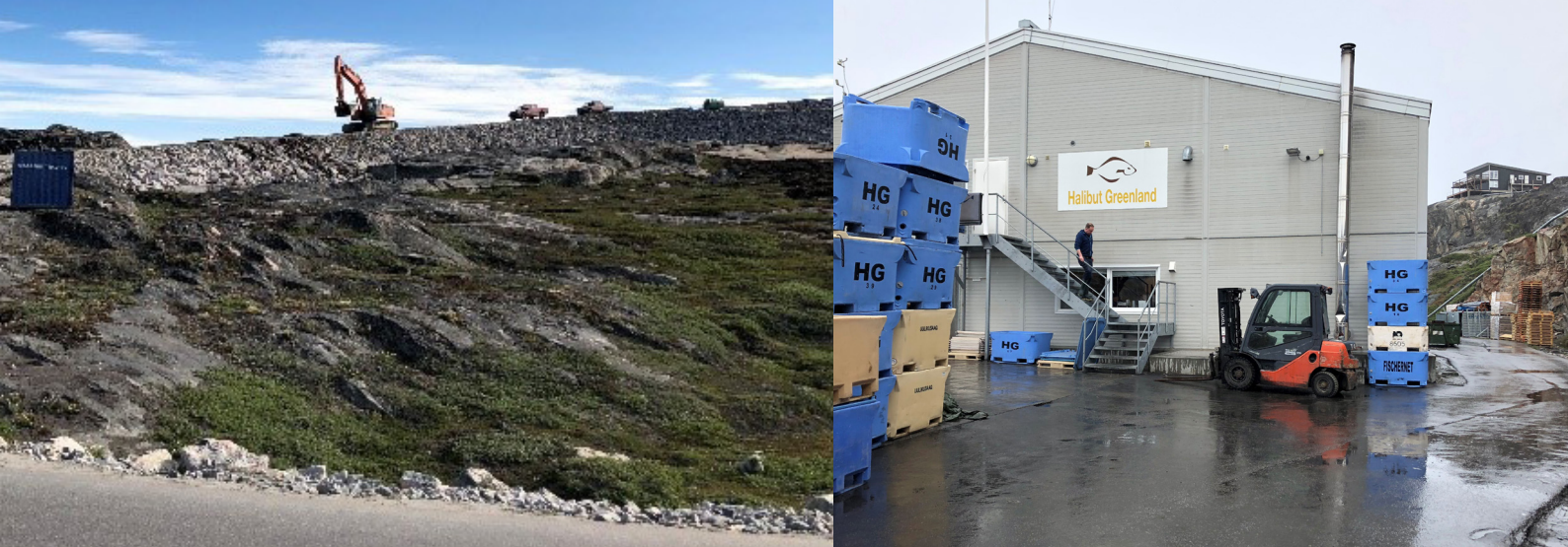
Construction in Ilulissat; the Halibut Greenland company. Photos: Karen Refsgaard
